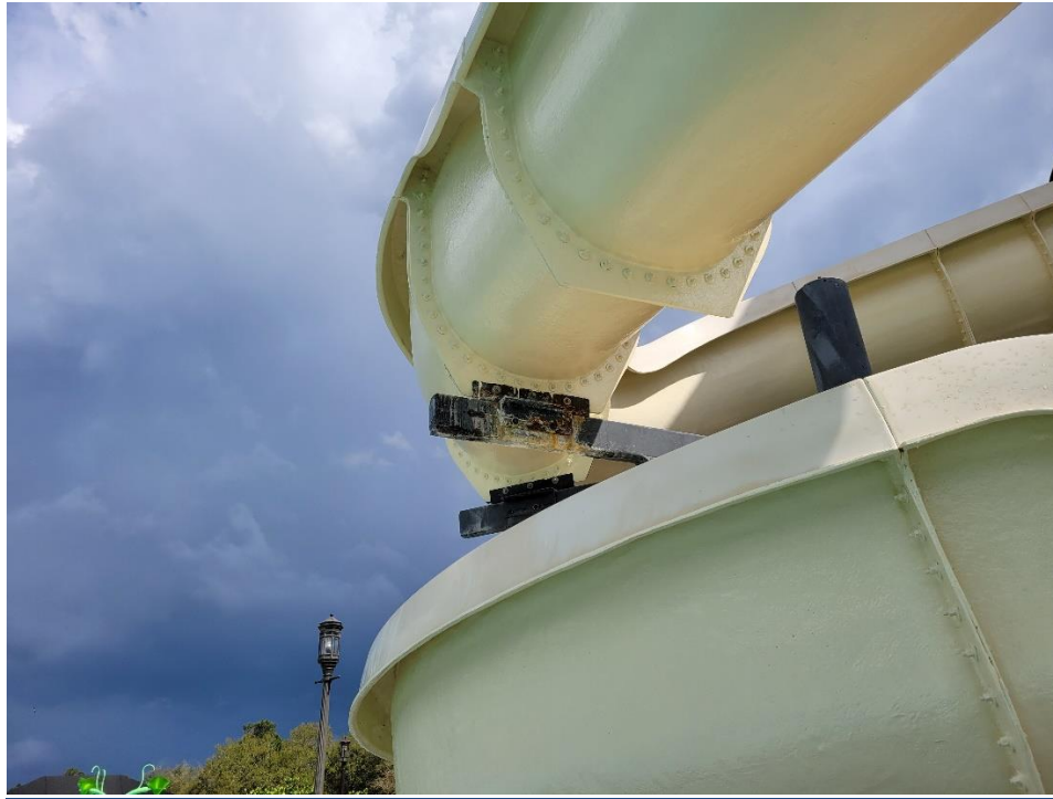
Photo 13: Corrosion of structure and connection at slide support
