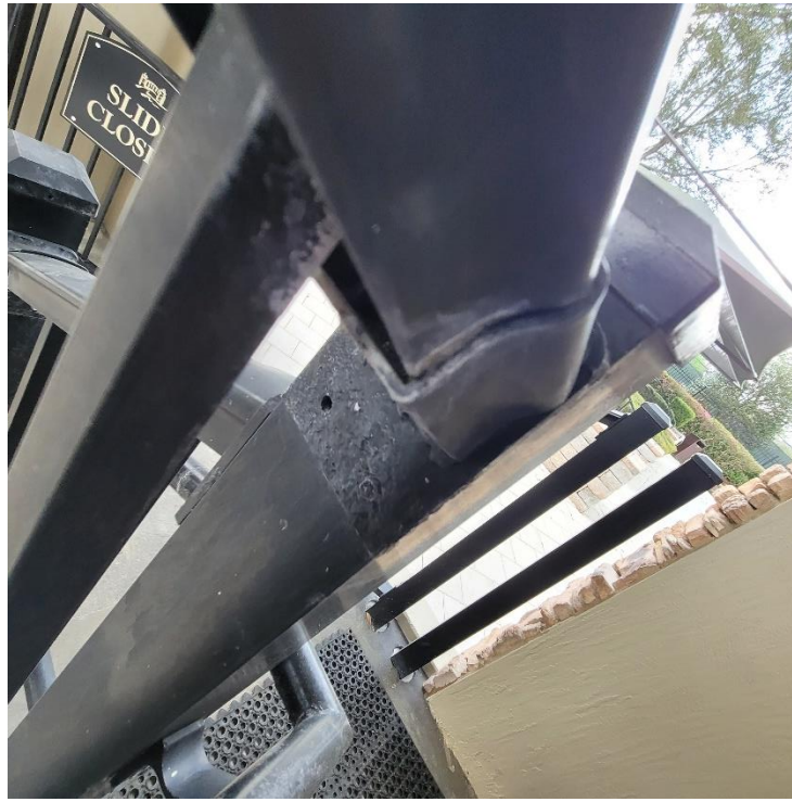
Photo 1: Bolt/screw missing at handrail bracket to post.
