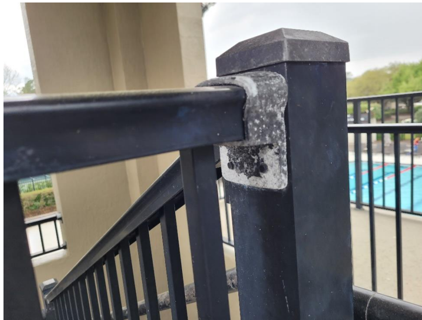
Photo 2: Deteriorating handrail to post bracket
