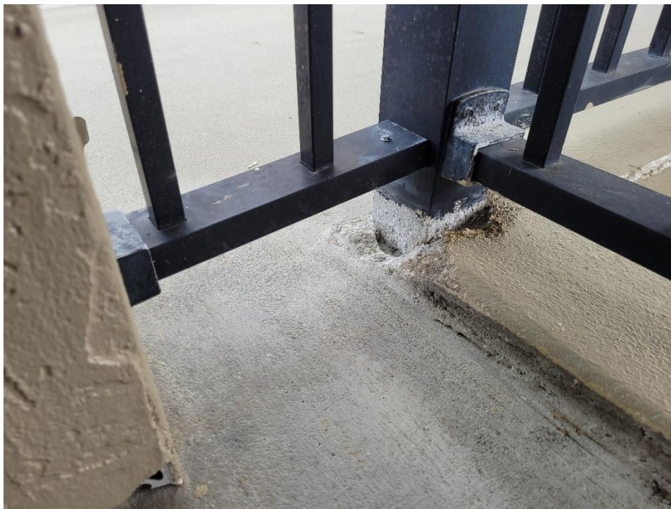
Photo 10: Concrete curb chipping away
