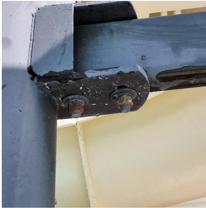
Photo 17: Oxidation of bolts and flaking paint at brace brackets
