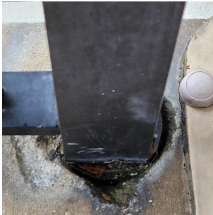
Photo 4: Grout pocket at handrail post missing
