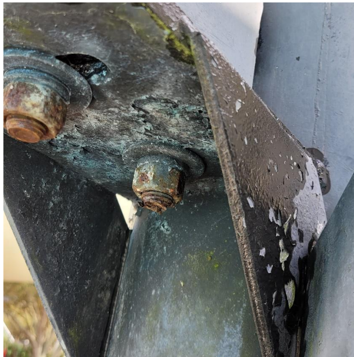
Photo 16: Oxidation of bolts and flaking paint at brace brackets
