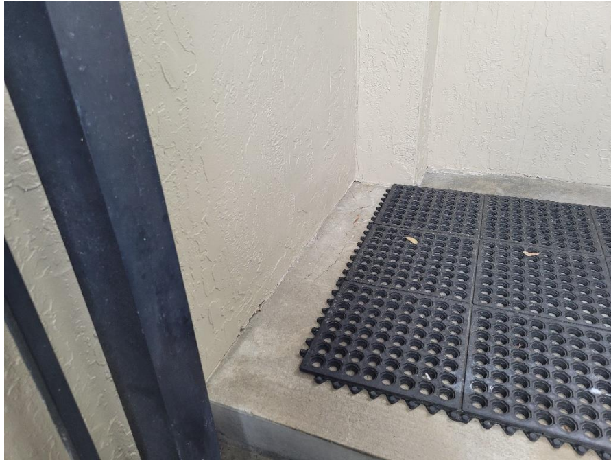
Photo 5: Concrete flaking/spalling at landing
