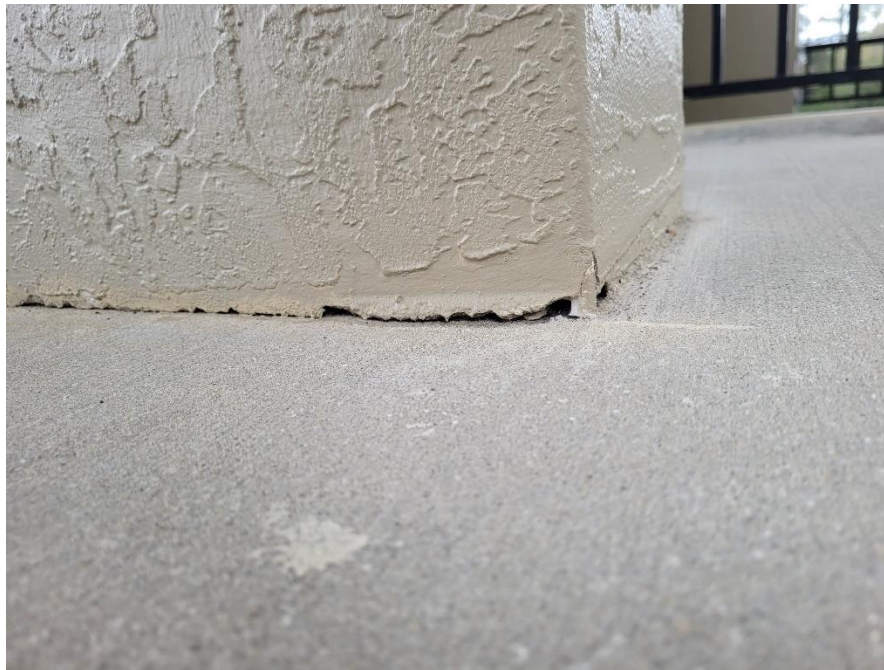
Photo 8: Sealant at stucco/slab/structure interface deteriorating
