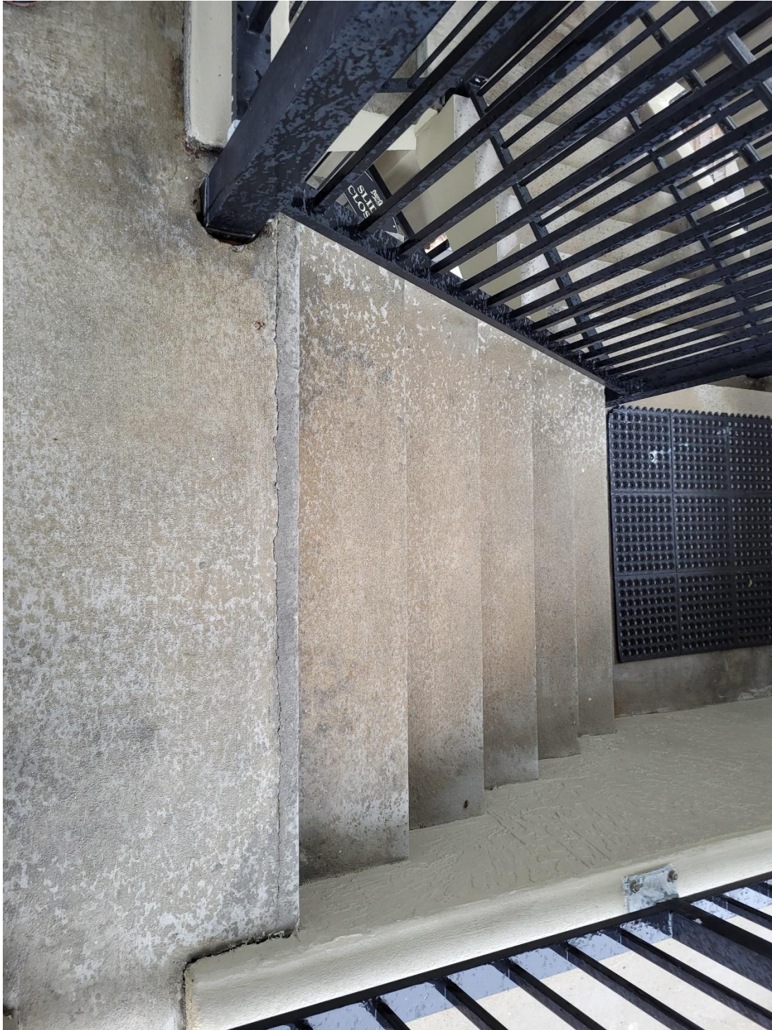
Photo 12: Crack in nosing up step
