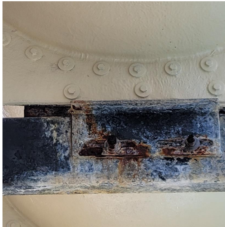
Photo 14: Corrosion of structure and connection at slide support
