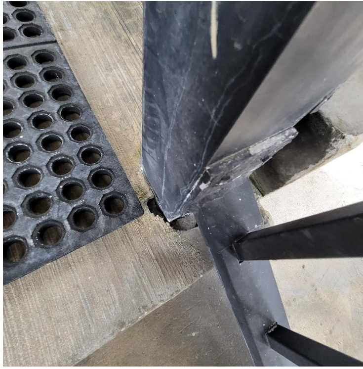
Photo 3: Grout pocket at handrail post base missing
