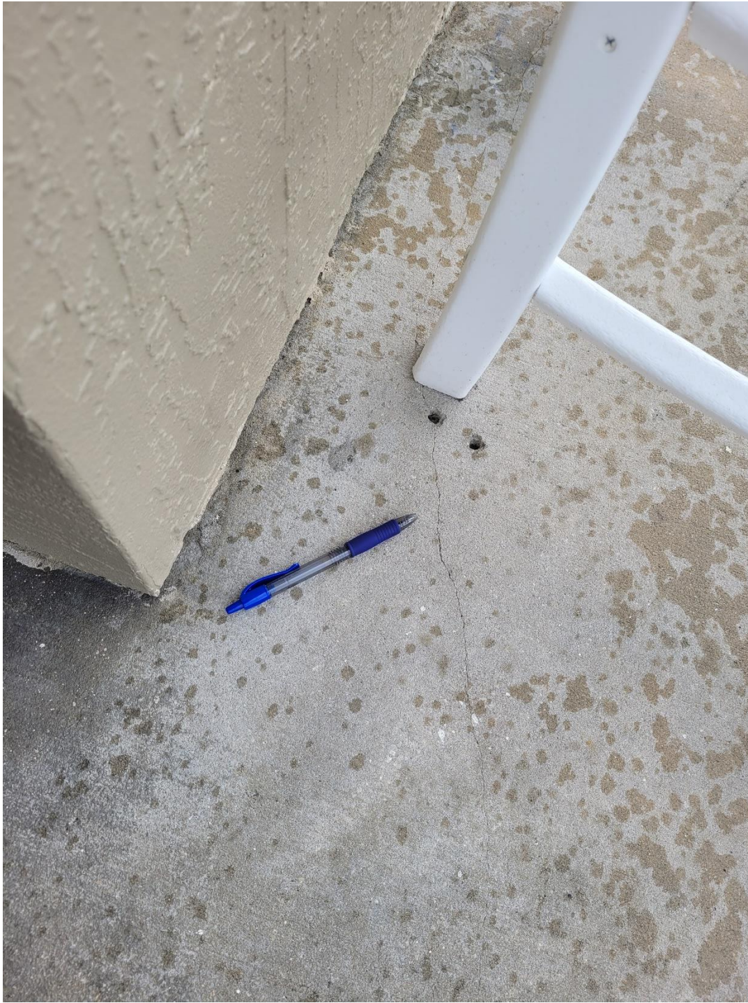
Photo 11: Hairline crack in upper landing slab
