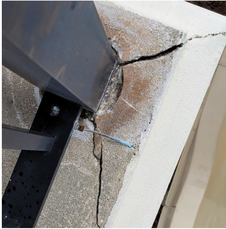
Photo 7: Cracking in upper landing slab
