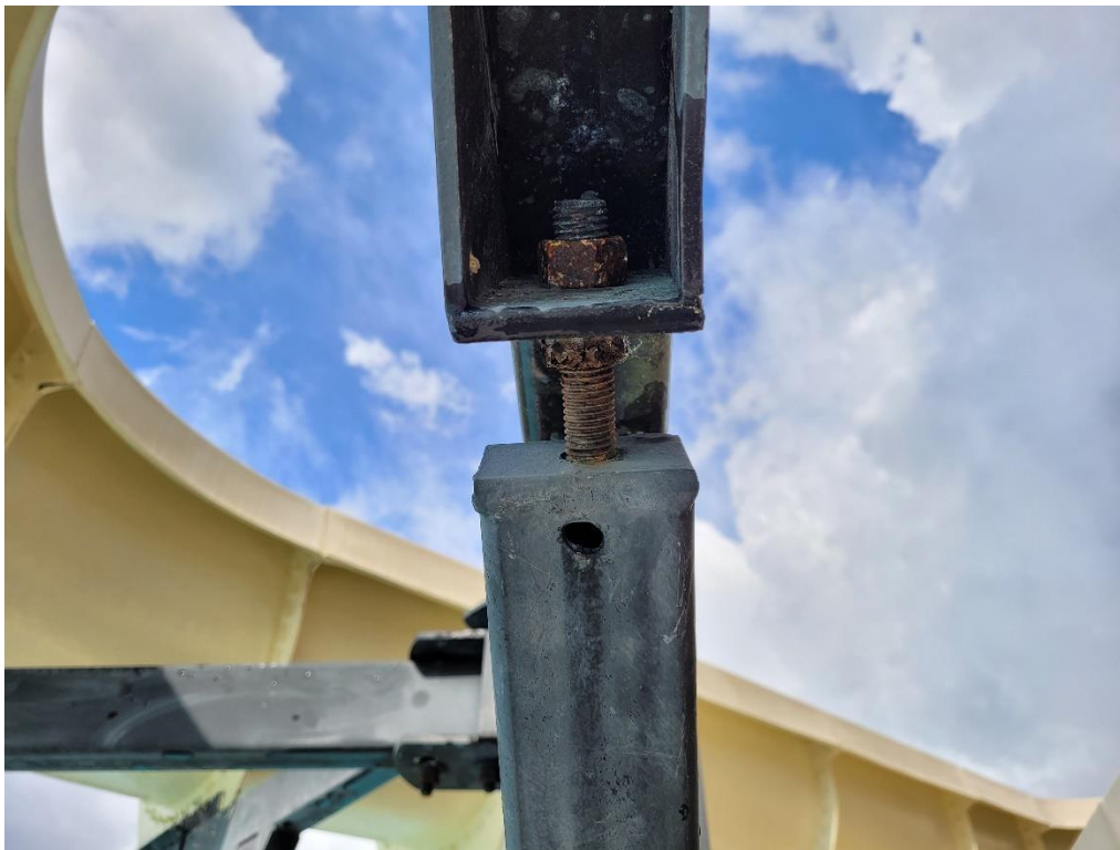
Photo 18: Oxidation of bolt in slide support brace
