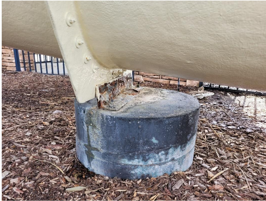
Photo 15: Corrosion of structure and connection at slide support
