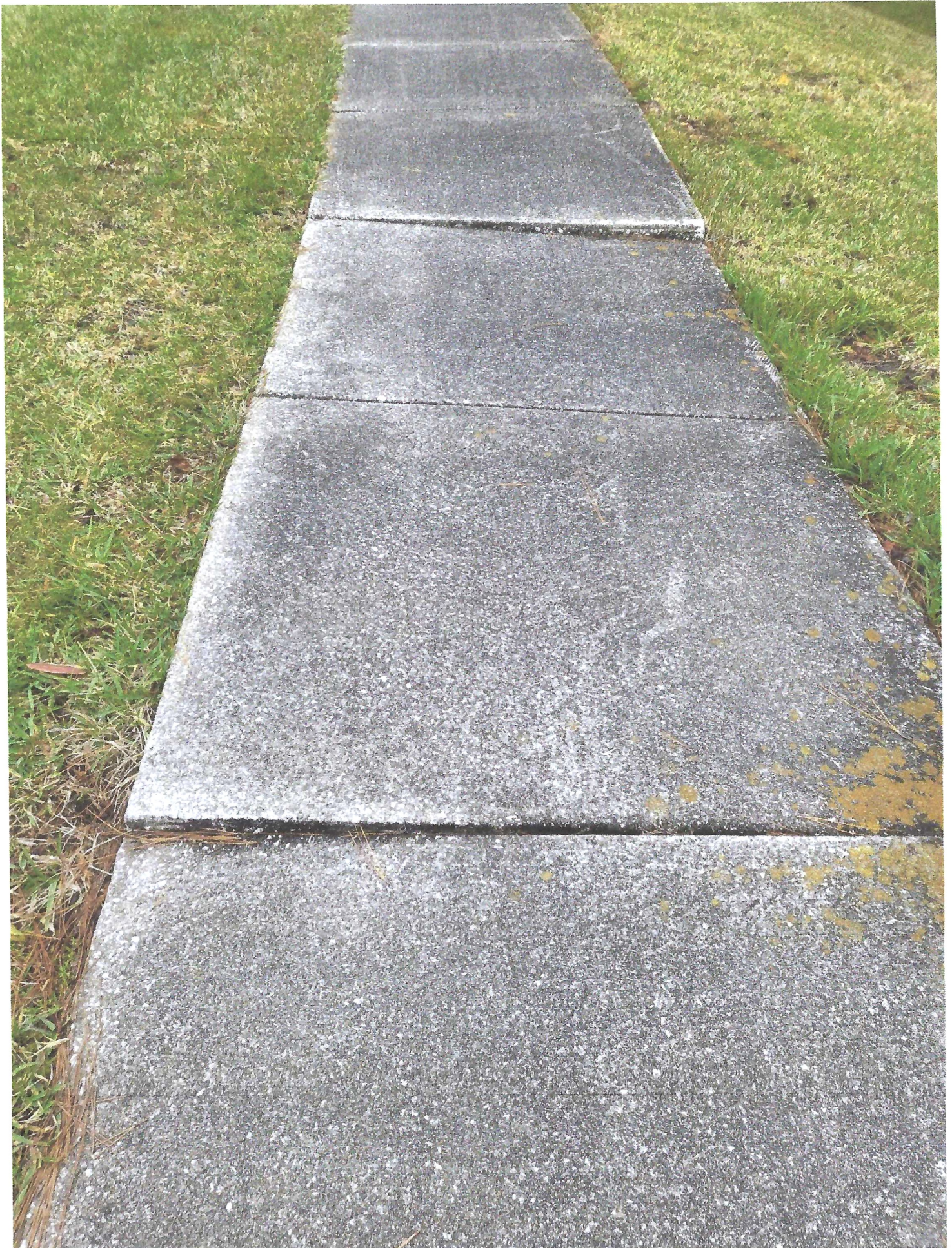
Leo Maguire sidewalk repair
