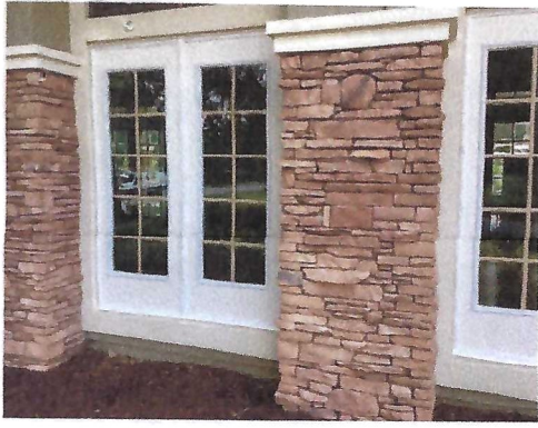
New Windows On Exercise Roo... Exterior Views of Windows
