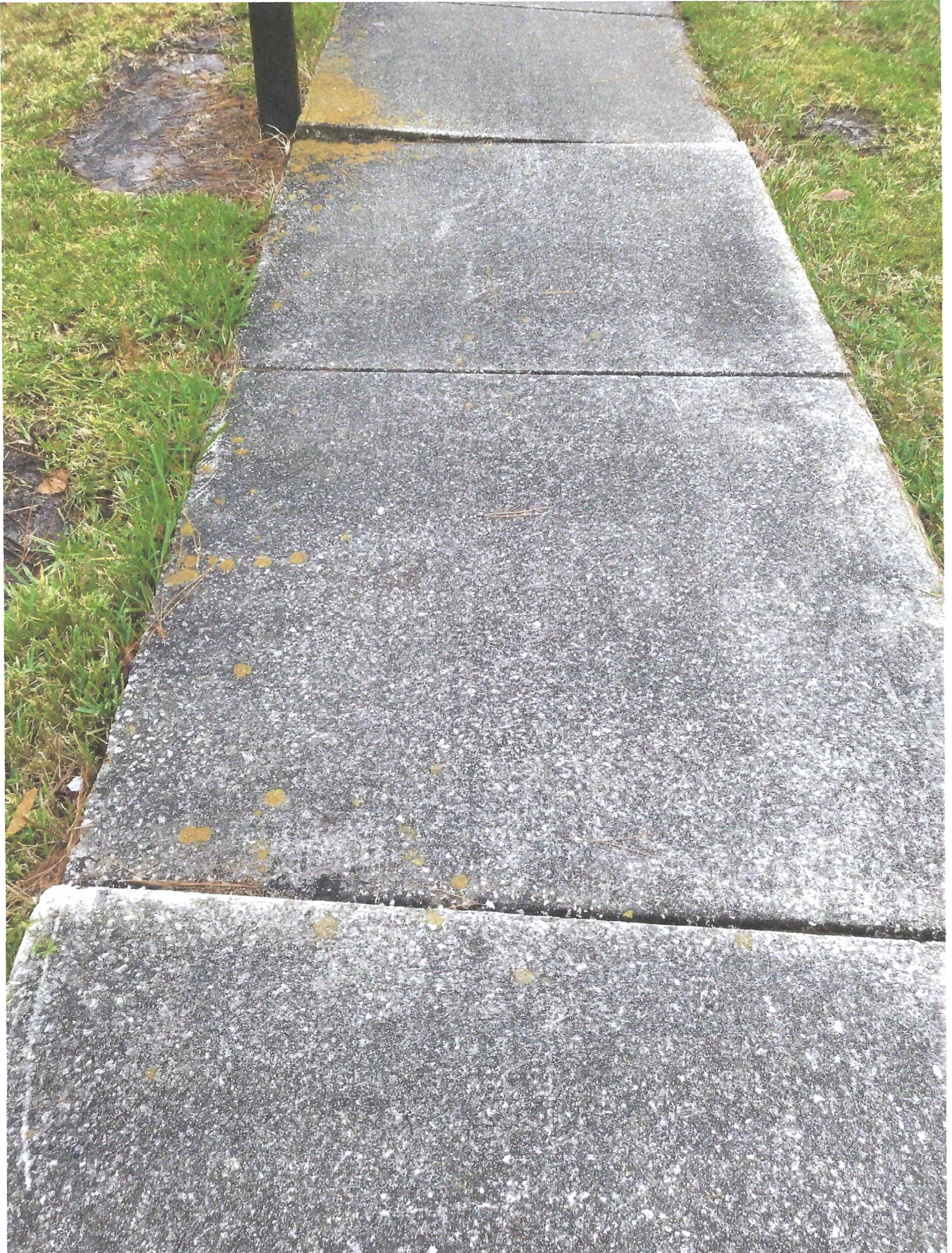
Leo Maguire sidewalk repair
