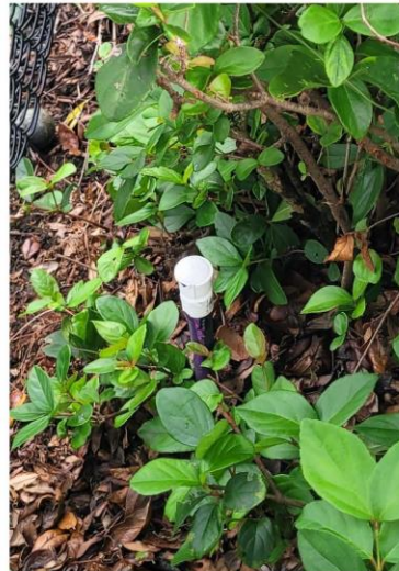
Adjusted and capped off sprinkler heads to prevent water on Tennis Courts
