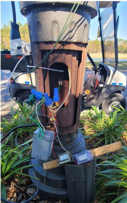
Transformer replacement for Holiday lighting.
