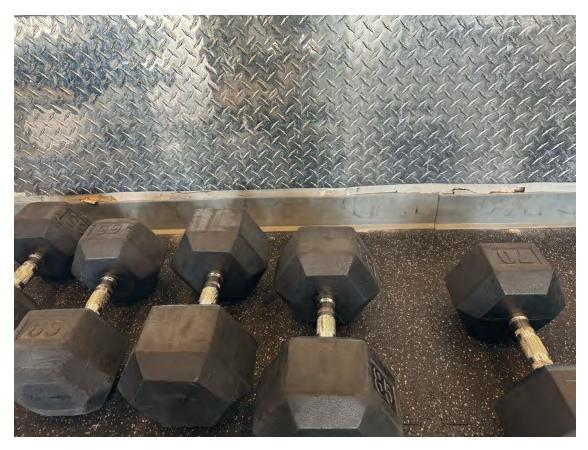
Figure 2. Damaged wall caused by dumbbells being placed on the floor and hitting into the wall.
