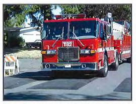
A speed cushion is placed longitudinally in the travel lane. Vehicles with wider axles straddle the cushion.
