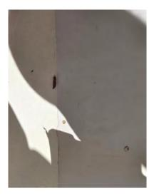
Flume 11 - Chipping and positive profiles on a previous repair - safety hazard
