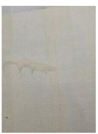
Flume 8 – The present seam repair has a high profile on which could cause scratches to the rider – Safety hazard
