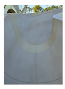
Flume 12 – High profile on a previous repair. This could cause scratching to the rider – safety hazard.
