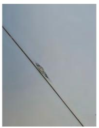
Flume 24 Start tub - Fiberglass crack on the start tub. If left unrepaired, condition will worsen.
