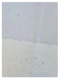
Flume 13 – High profile on previous repair that could cause scratching to a rider – safety hazard. Resin chipping on the exterior of the should which will cause water intrusion, causing the fiberglass to weaken.
