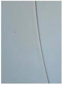
Flume 16 – Present spider crack and should be repaired. Gel coat burn spot was found and crack should be repaired – Safety hazard.
