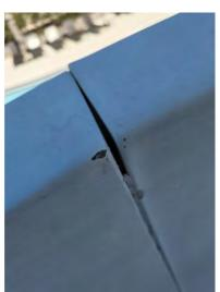
Flume 15 – Spider cracking and a stress crack in the fiberglass – cracking causes water intrusion which causes the fiberglass to weaken – safety hazard.
