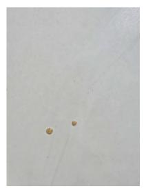
Flume 20 – High profiles on previous repair could cause scratching on riders – safety hazard.
