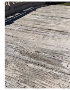
Close up on wood condition
