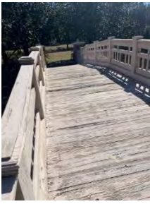
Overview of Bridge
