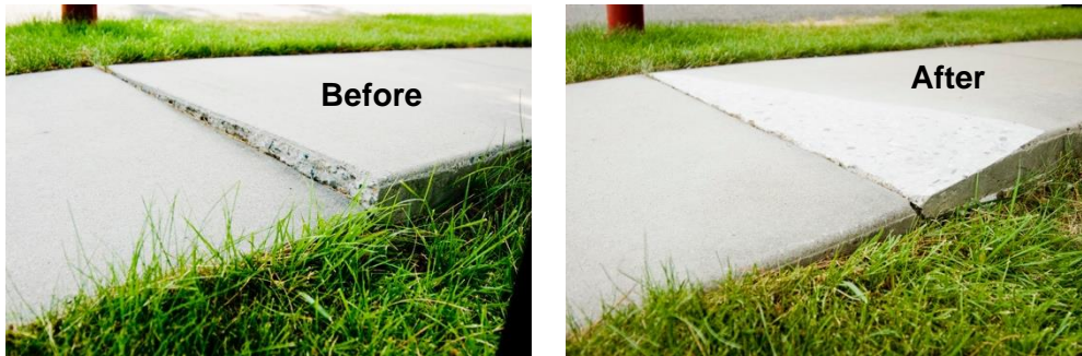
Figure 10: Precision Sidewalk Safety Work Example
