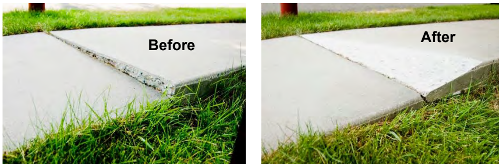
Figure 11: Precision Sidewalk Safety Work Example
